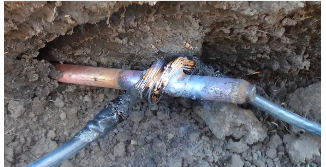
Brazed Rod Connections
